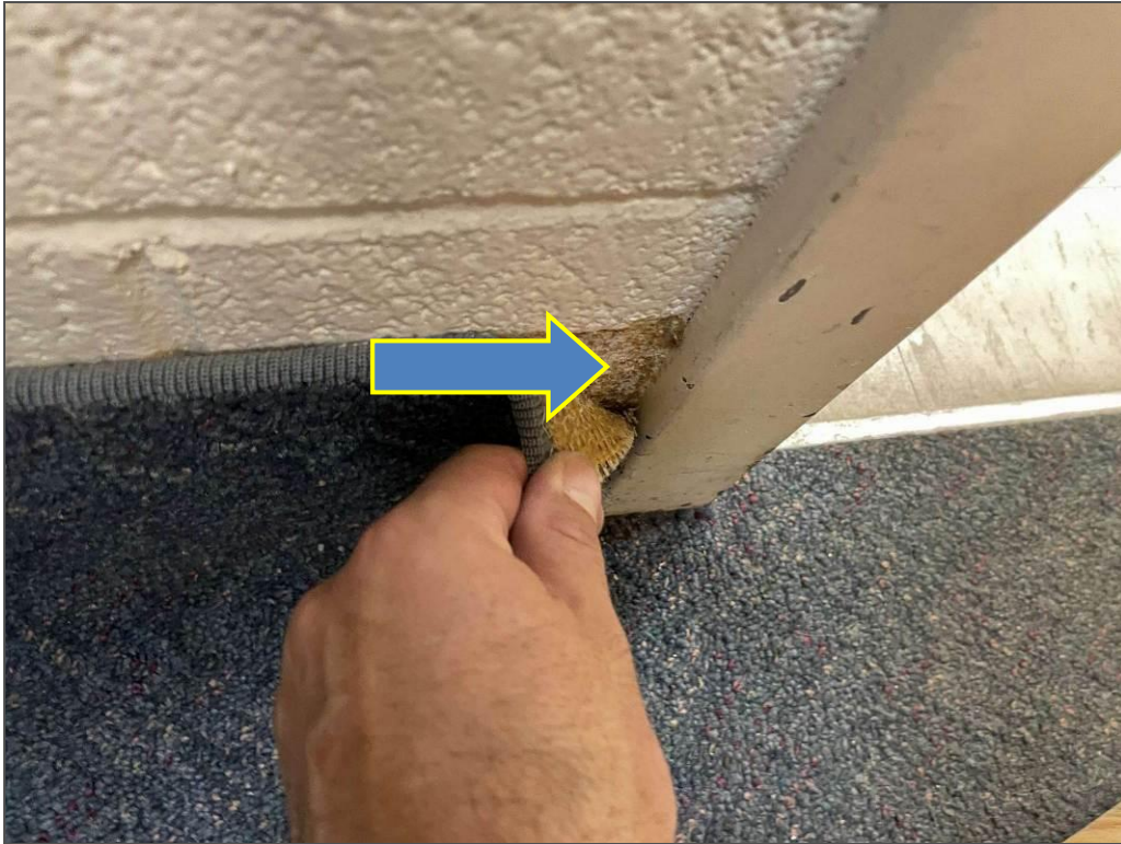
S1103A (None), Brown behind carpet baseboard, Wall, Base, Mastic, Office (Location #: 320)
