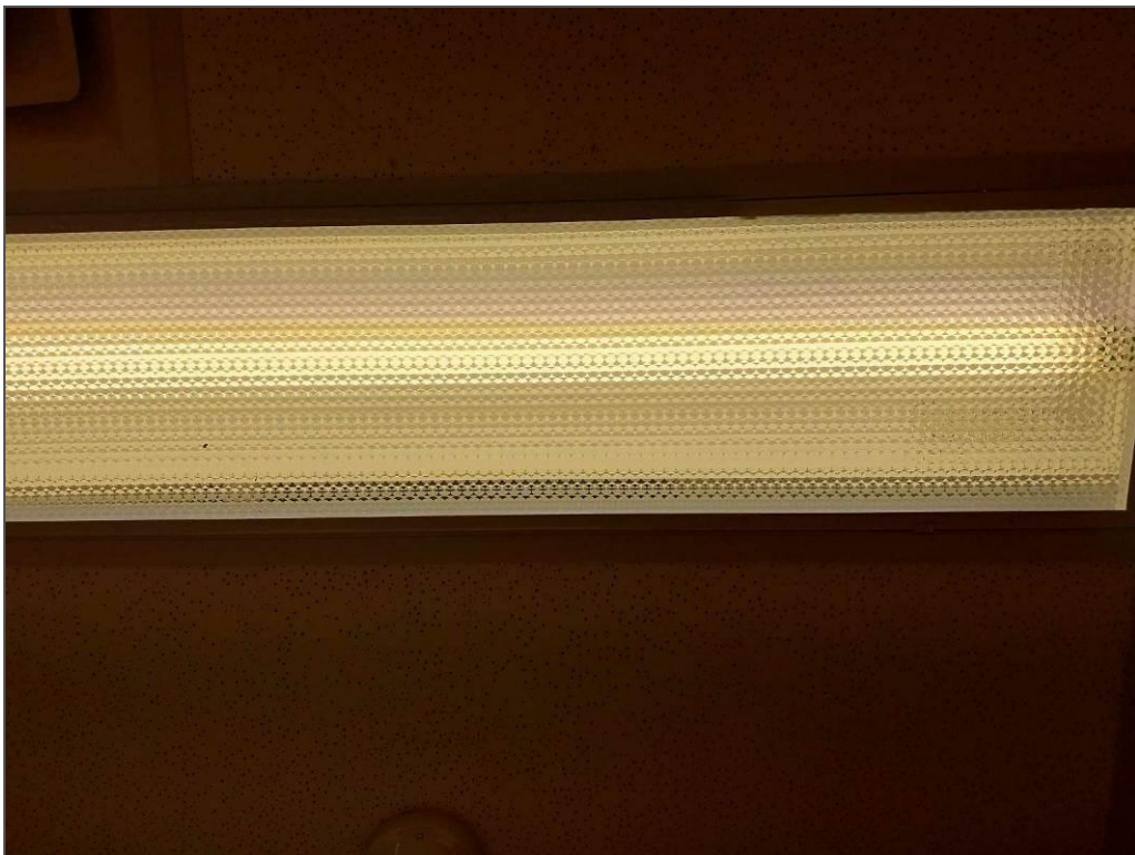
Mercury, V9500(Presumed), Light Fixture, T8, File Storage (Location #: 39)
