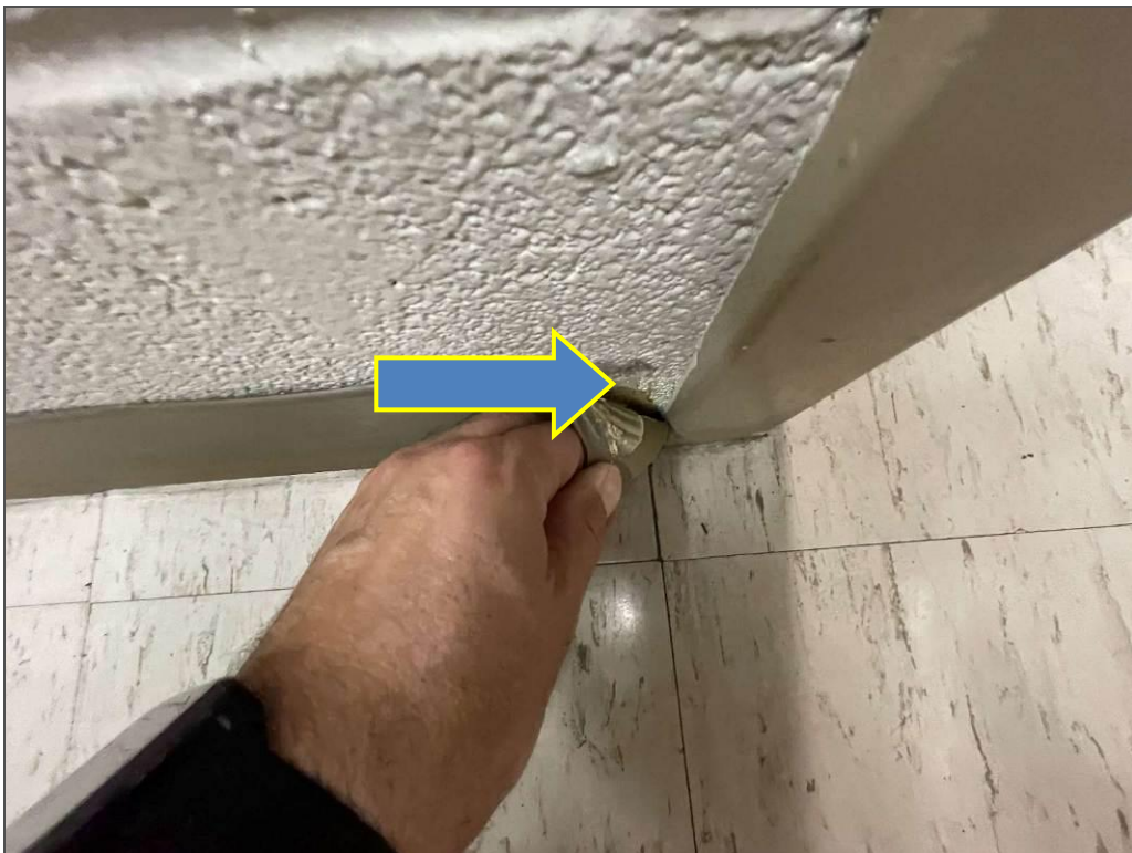
S1104B (None), Brown mastic behind rubber baseboard, Wall, Base, Mastic, Central Dispatch (Location #: 37)
