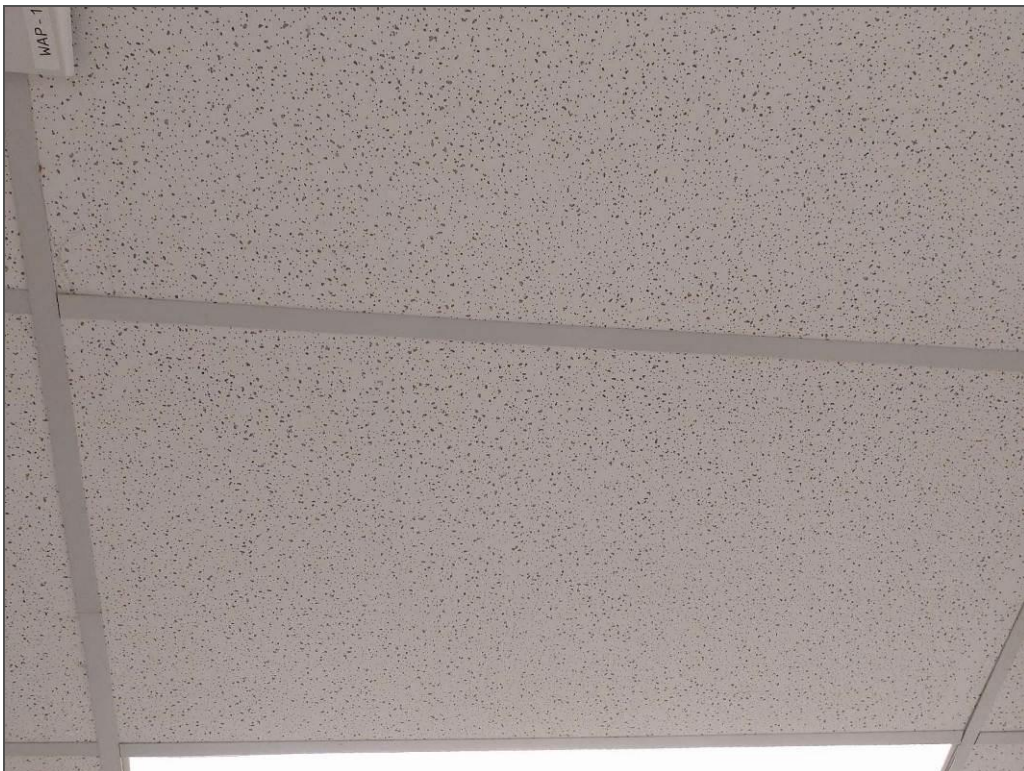
V0000 (None), 24"x48" pinhole and fleck, Ceiling, Ceiling Tiles (lay-in), Central Dispatch (Location #: 37) 2007 date stamp
