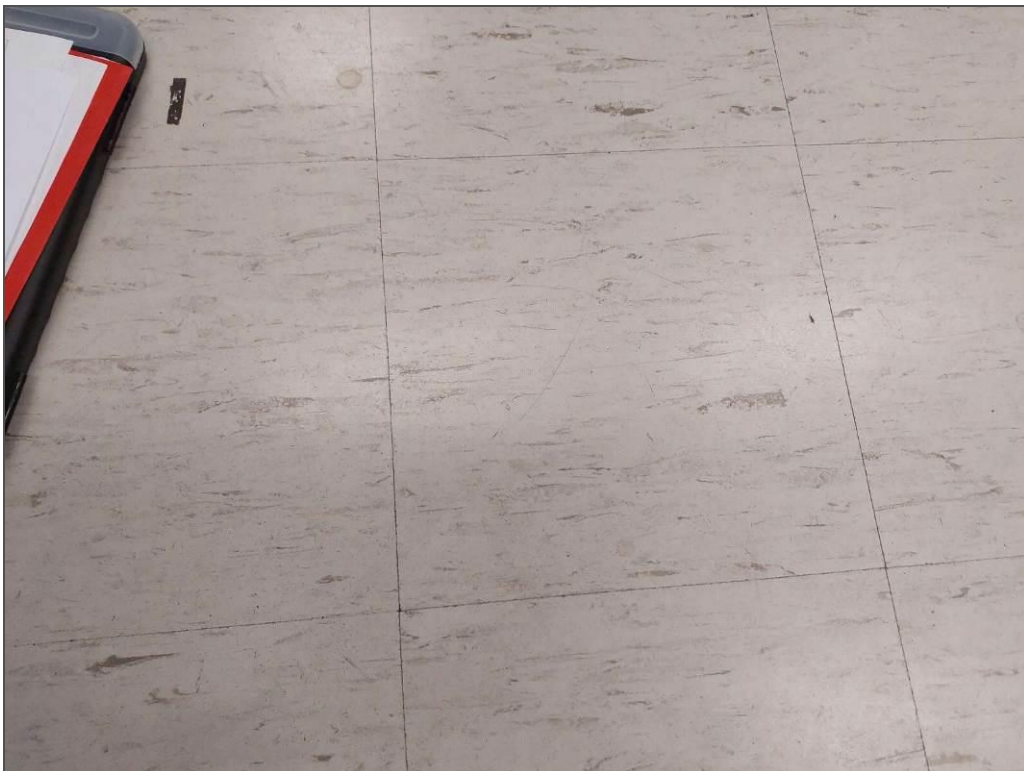
S1101A (Confirmed Asbestos), 12"x12" grey with grey streaks, Floor, Vinyl Floor Tile and Mastic, Pharmacy (Location #: 38) Possible 23
