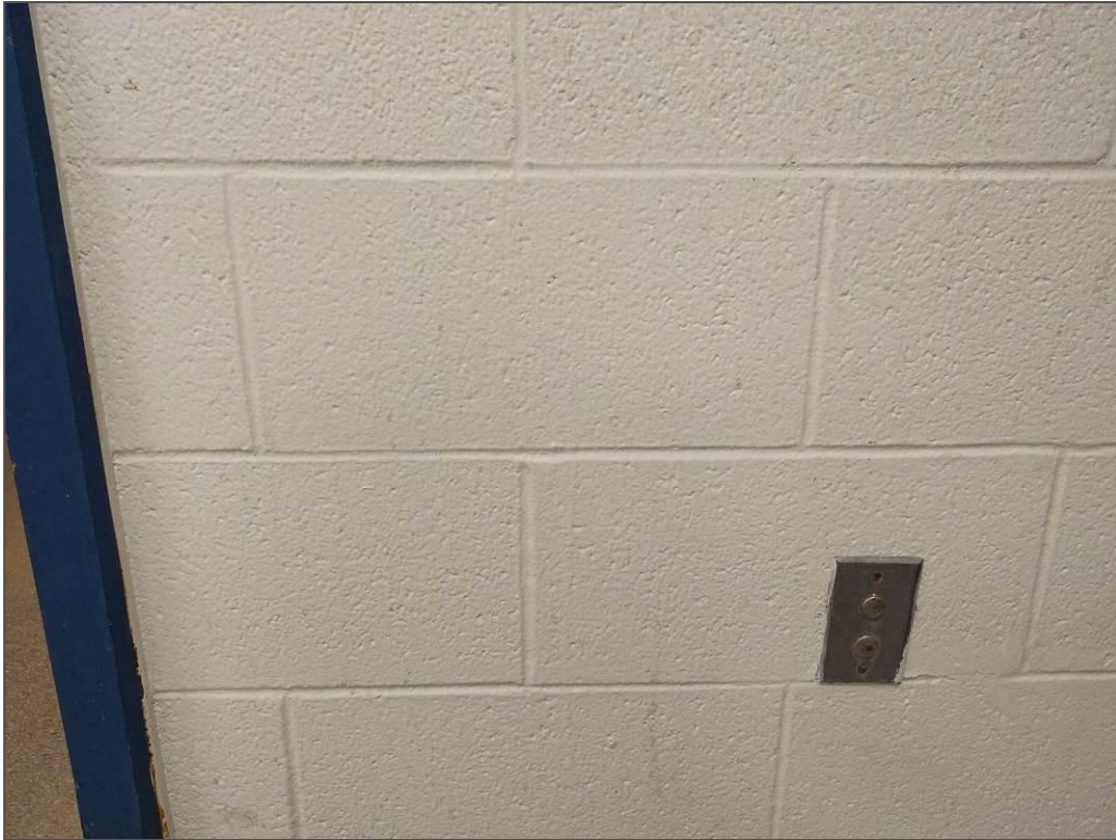
L0018(Lead, None), Paint on block walls, Wall, Dishwashing Area (Location #: 318)
